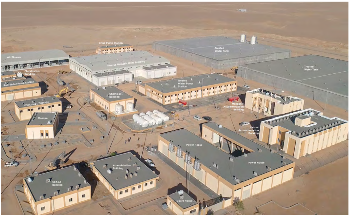
Layout of the Al-Wajeed Water Treatment Plant.
