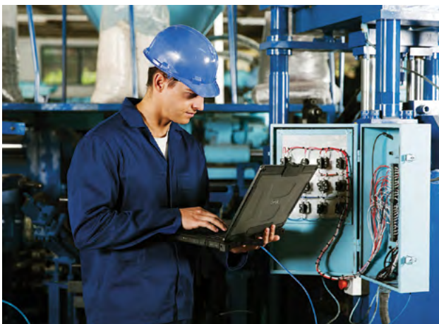
Equipped with rugged laptops and the powerful processors of these devices, workers can more easily collect, process, and transfer data and information quickly, thereby eliminating manual data entry entirely.
