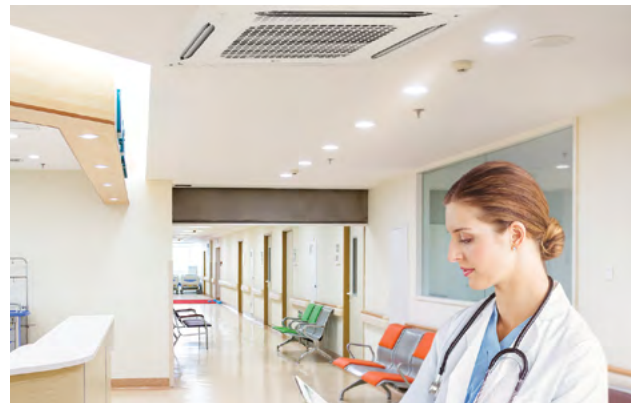
Indoor air purification panel installed on ceiling
